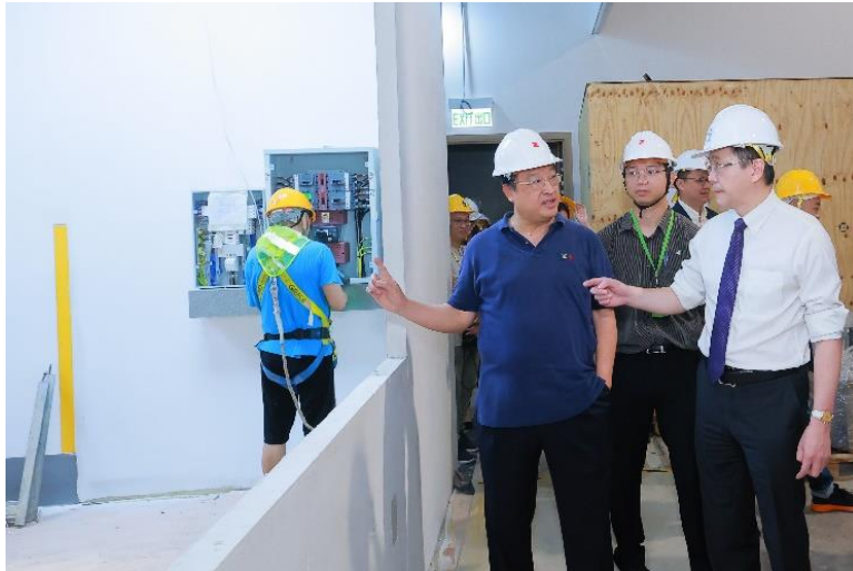
Photo 2: Accompanied by Dr Alex Wong, Director of Nanoshields Technology (front row from the left), Professor Sun Dong (front row from the right) visited Nanoshields' electrospinning production lines for nanofiber material under construction.
