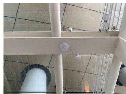
(b) A wifi sensor installed at the Atrium Link @ Hong Kong Science Park (Source: Prof. Gary Chan, HKUST)
